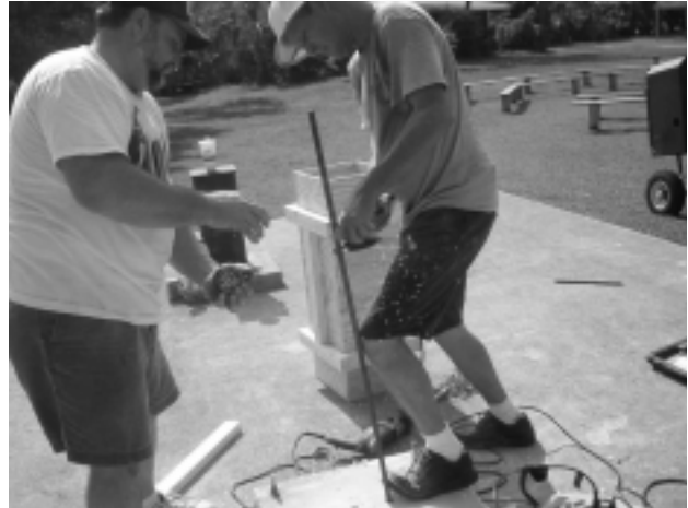
Nick (L) and Steve (R) cut rebar to the correct length.
